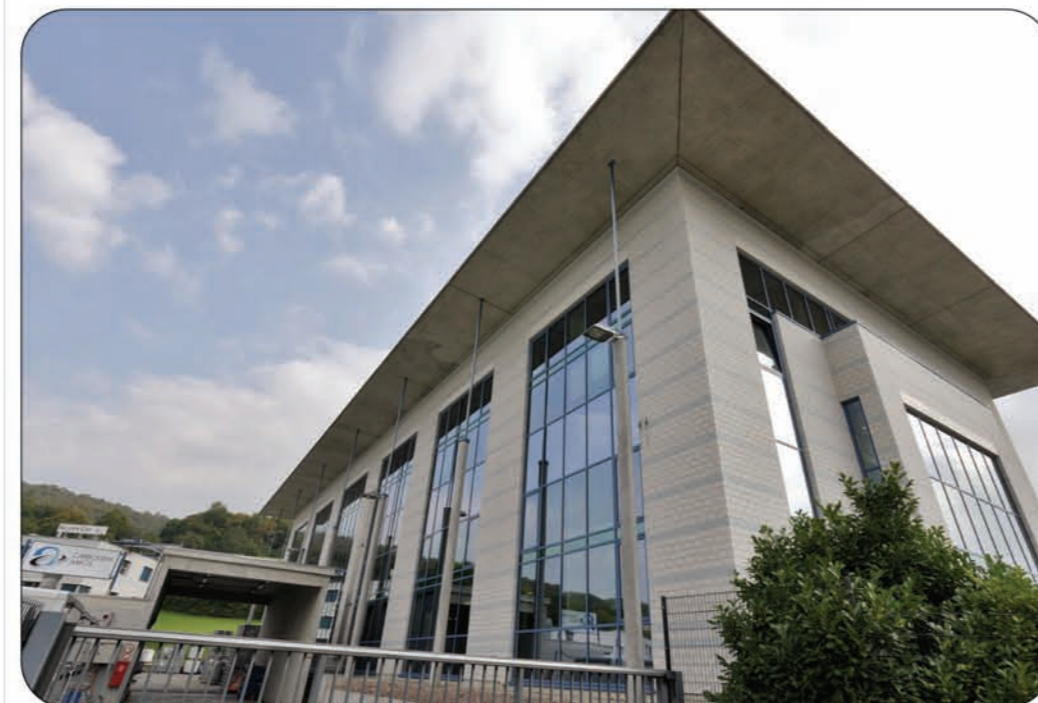
API manufacturing facility (Bubendorf).
