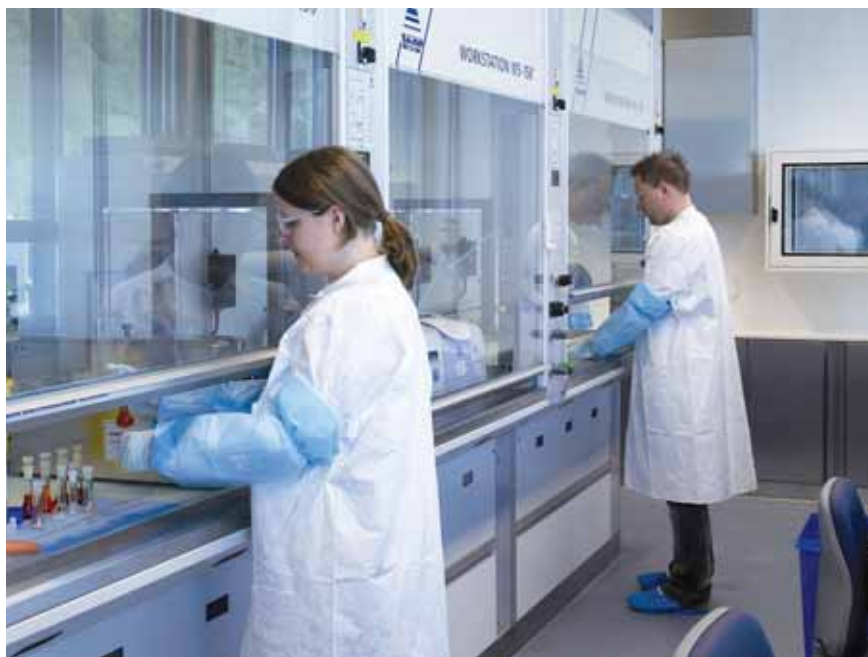
The sample pass-connected and flow-controlled Skan-hoods in Carbogen Amcis' analytical lab for HiPo APIs; a material airlock can be seen at the back
